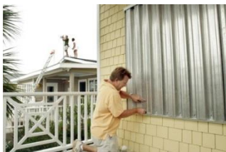
Shutter Installation & Removal
