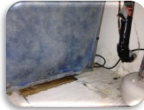
Water Heater & Air Handler Leaks
