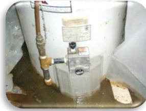
Water Heater & Air Handler Leaks
